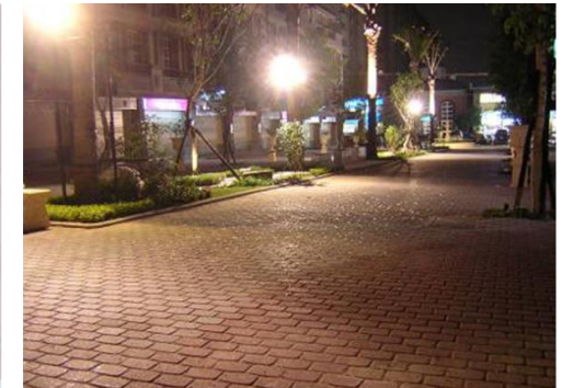
Commodity Name: Sandblasted Colored Spar Floor Tiles Feature Introduction: Ranging from \Phi 1 to 3.5 mm, these tiles are formed by combining high-pressure vibration and exposing the surface layer particles through sandblasting. Applicable Objects: Ideal for various public facilities.
